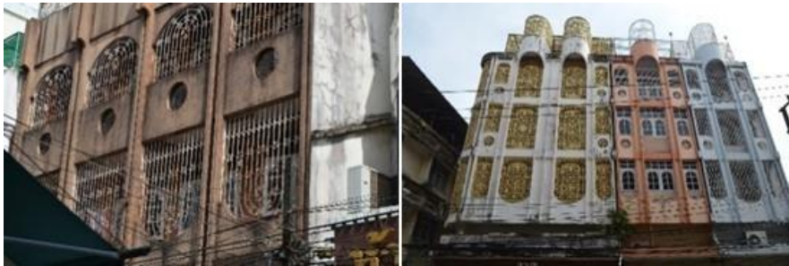
Figure 3. Patterns of Wrought Iron in Modern Building Styles of Chanthaburi
