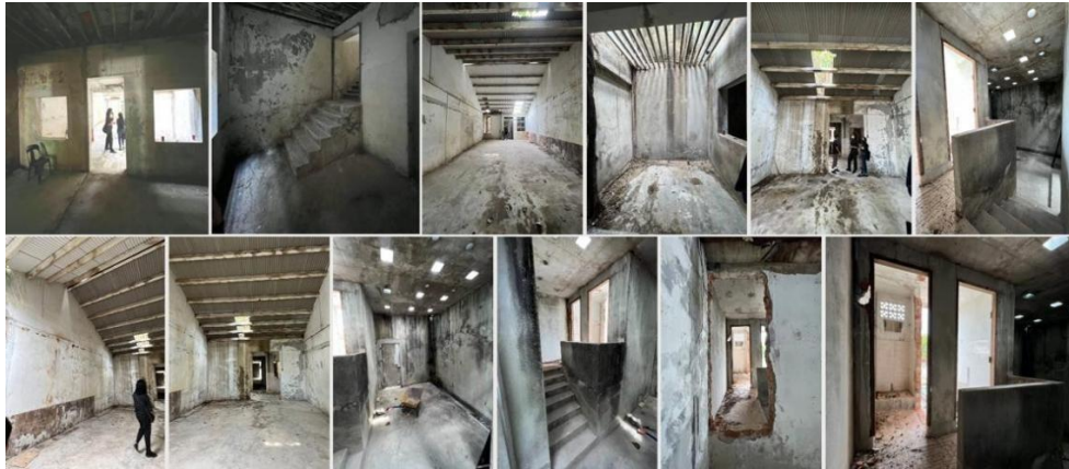
Figure 2. Images of The Ground Floor Condition Before Renovation
